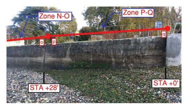
Photo 2. South Portion of Seawall. Source: Reid Middleton Site Visit 10/18/2016 Note: Dimensions roughly field measured – for assessment purposes only.
